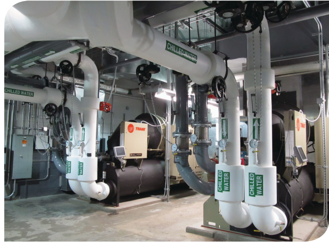
Water-cooled CenTraVac™ chillers with variable frequency drives increase reliability and energy efficiency.
