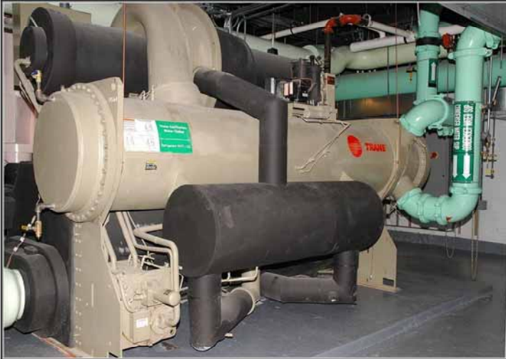
One of three 800-ton Trane chillers part of a thermal storage system.
