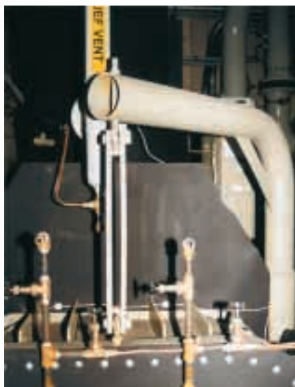
Chillers were ordered with gantries to facilitate removal of waterbox covers for inspection and tube cleaning.
