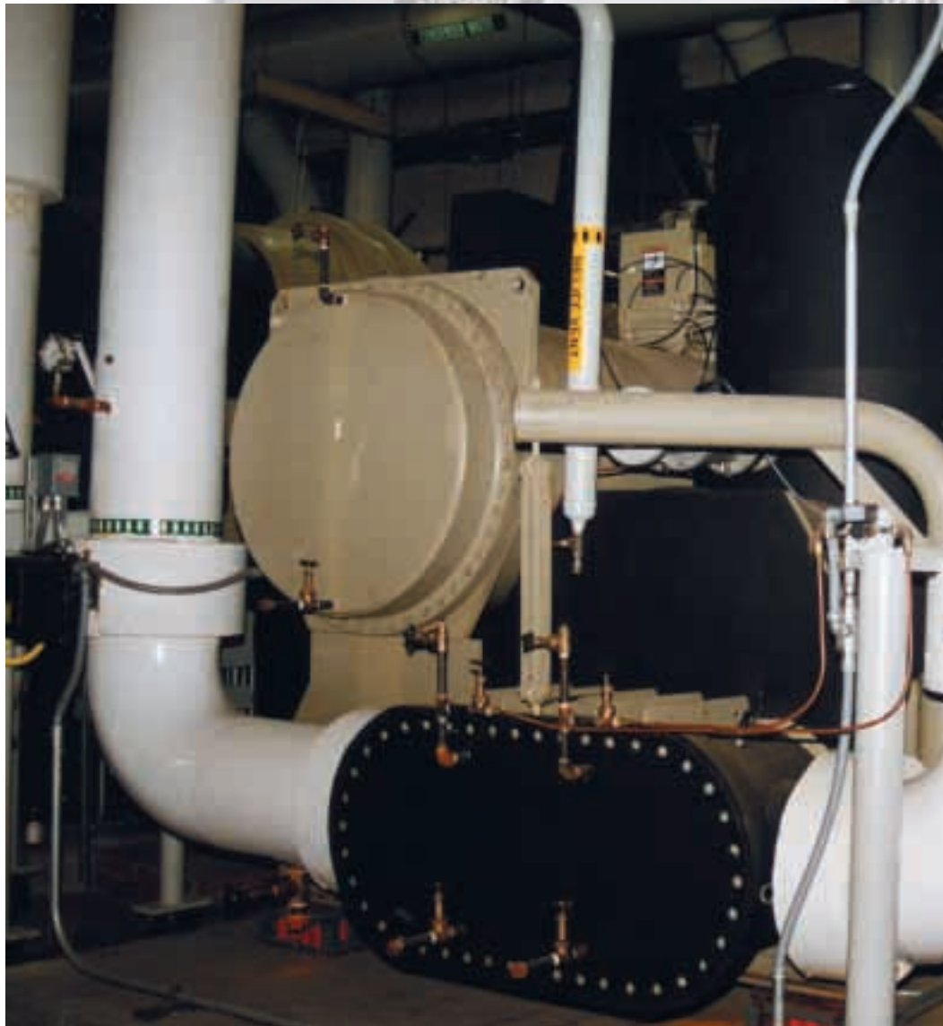
Three 1,100-ton Trane Model CVHF two-stage centrifugal chillers running on HCFC-123 with new piping, pumps and remote indicator panels to monitor status replaced the old steam chillers.
